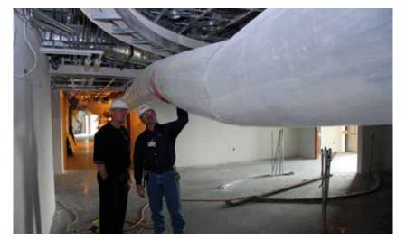
A flexible air distribution system was woven through stairwells and floors to reach all areas that required humidity control.
