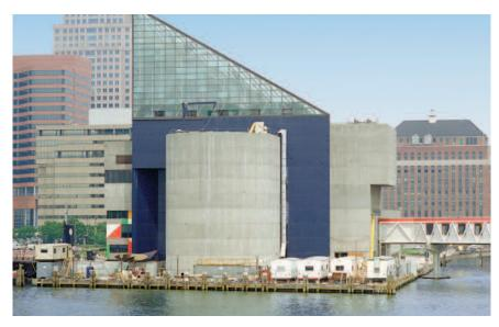
Handling a difficult site problem – normally, large dehumidifiers would have been used to dry the 130,000 cu. ft. tank at Baltimore's National Aquarium, but limited on-site space required a more flexible solution. Polygon's versatile fleet provided combinations of lighter and smaller dehumidifiers which could be positioned in available locations.
